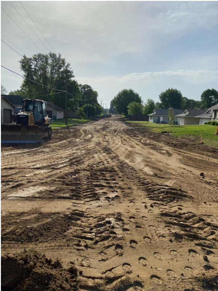
Above: Completed utility installation along the east end of Midland Avenue.
