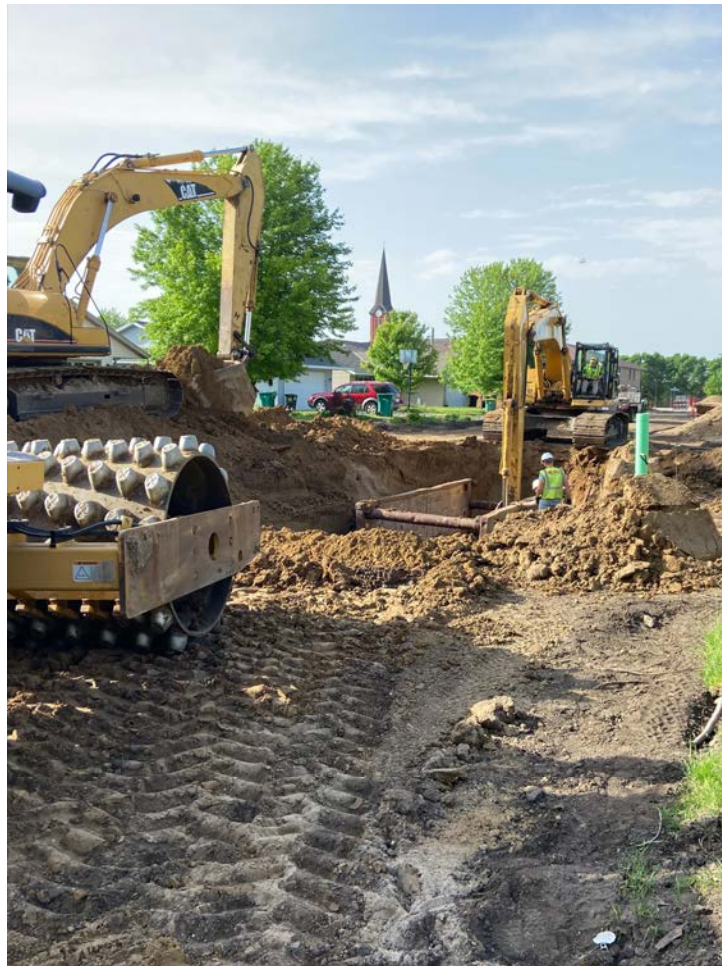
Left: Breitbach Construction installing sanitary sewer main along 3rd Street.
